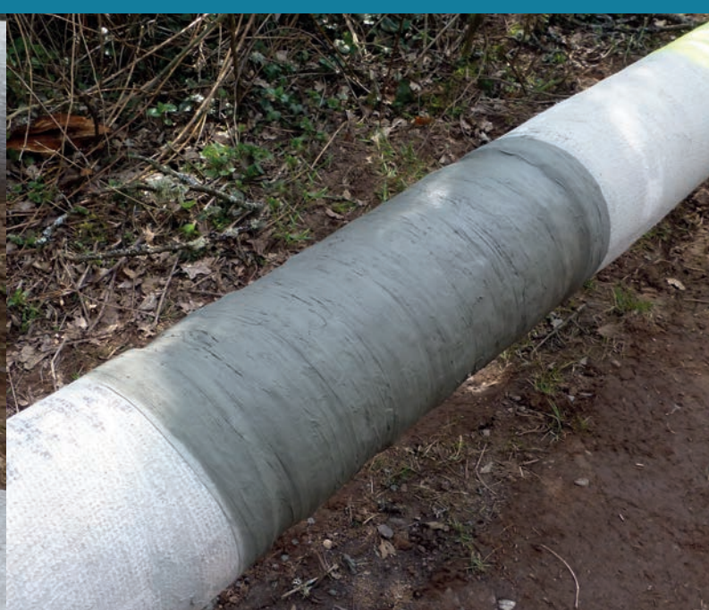
WELDED JOINT DN 150
