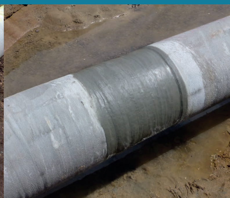
WELDED JOINT DN 500
